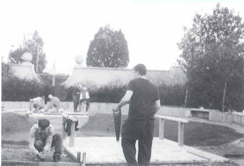
(Left) New Deal's Environmental Task Force in action building a pond
