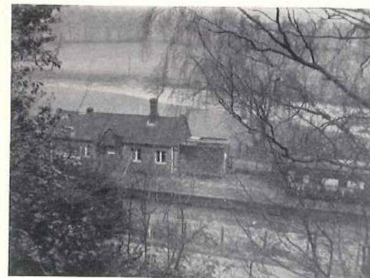
Kerne Bridge where rebuilding is now complete
