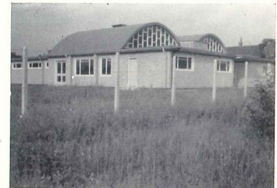
The Ramblers Lads Club in Gloucester nears completion
