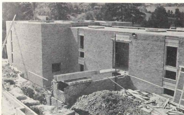
The New Boys' Club at Stroud nears completion
