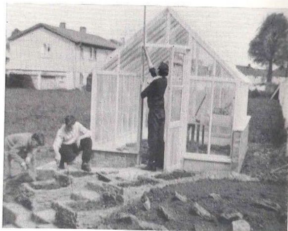
Whaddon and College boys build a greenhouse . . .
